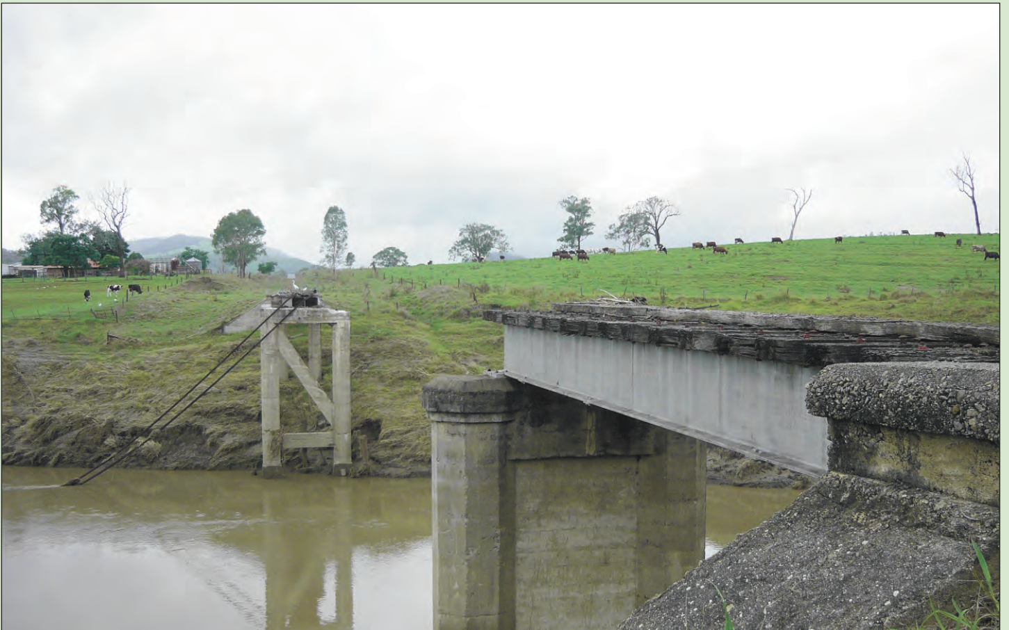
Below: Maronghi Ck bridge after the 2013 floods where three piers were washed out. It is not clear why the bridge did not survive this flood but its loss is obviously a major impediment to the development of this scenic section of the rail trail.
