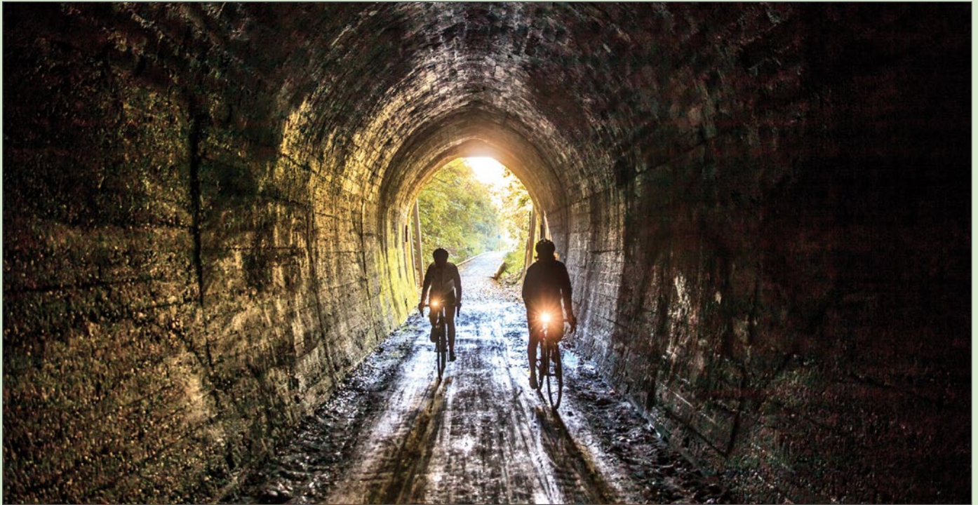
Lights are essential in the 1325m Spooners Tunnel opened in 1893. Photo: George Guille Media
